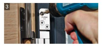
The inserted **MASTERBAND** FX2 120 3-D CS is screwed into the frame with standard screws. Mounting of the door element is now complete.
