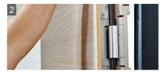
The door leaf is connected to the frame. Now, the hinges are inserted into the frame recess. An assembly dolly can serve as an aid or assembly cushions, wedges, etc. can be used.
